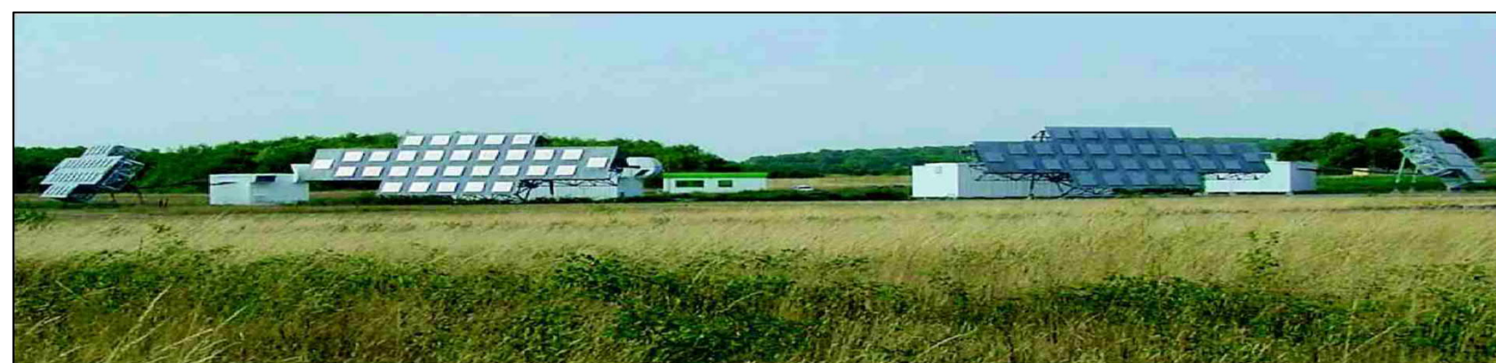
Fig. 4 The 143.050MHz GRAVES planar array antennas near Dijon, France.
